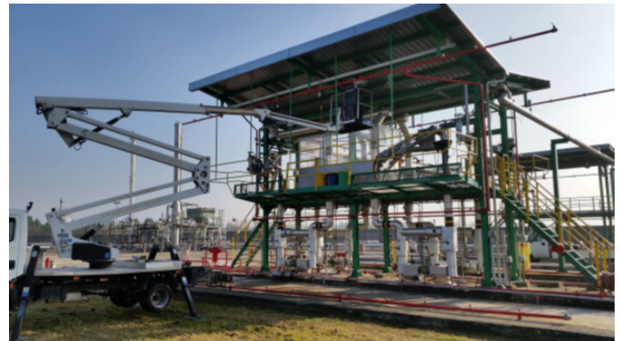
Example of installation of RAIL.
